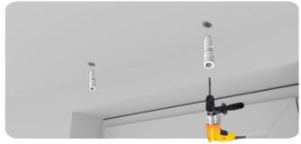
Stage III Screw the mounting hangers.
